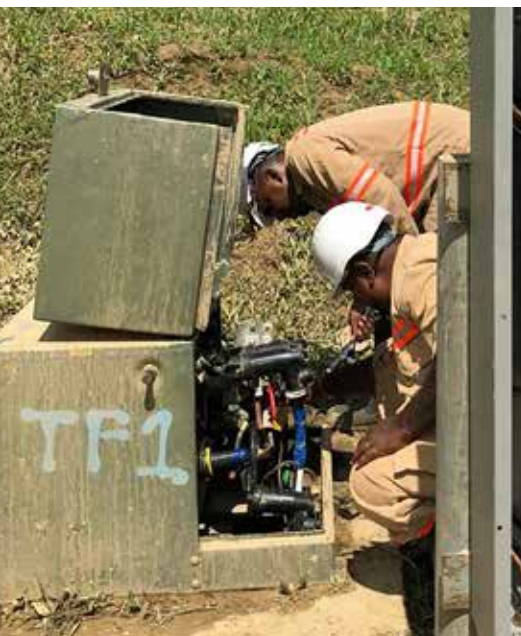
Employees at work to restore power to affected customers.
