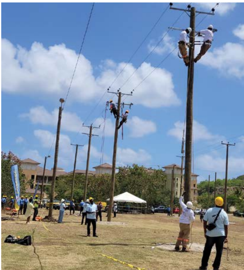
Competition time for the team (foreground) in the HT cutout installation event.
