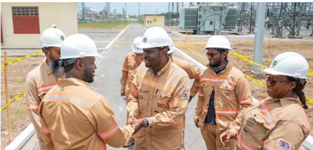
Minister of Public Utilities, the Hon. Marvin Gonzales, greets employees at the Union Substation, La Brea, after the ceremony to mark the commissioning of a second 220 kV double circuit tower line from Union Estate Substation to Gandhi Village Substation.
