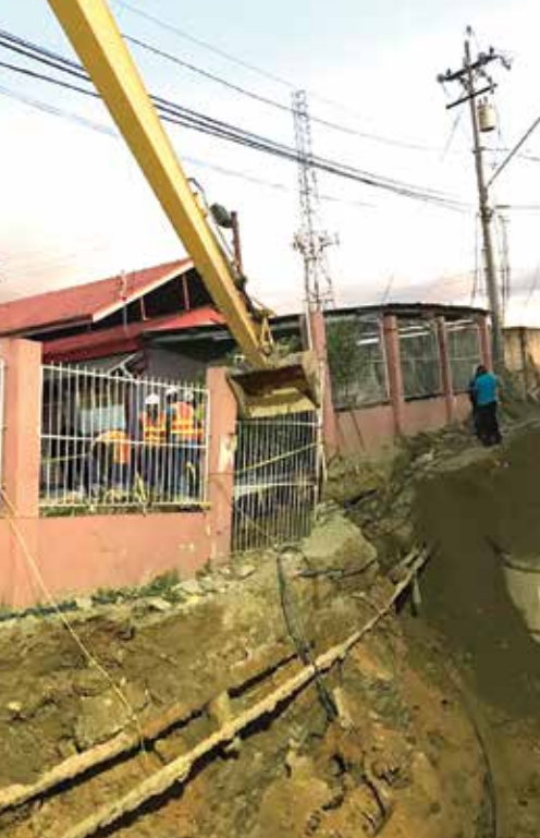
Excavation work being done to facilitate the installation of sewage pipelines in the Beetham area.
