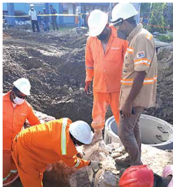
Senior Supervisor, Gairy Nelson, overlooks work being done by contractors to access the underground high-voltage cable in the path of the sewer pipeline installation (photo from WASA).
