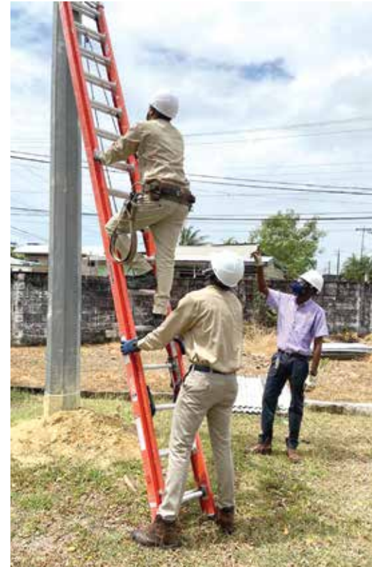
Instructor I, Kwame Chikuyu (right), guides Duane Heywood and Trent Trotman on how to secure an extension ladder on a pole at the El Socorro Training Facility.
