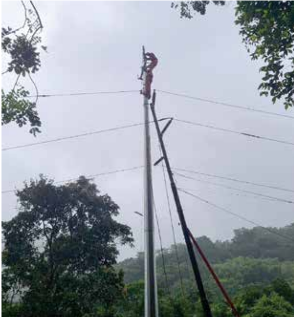
Employees perched atop the 21 meter pole being installed to replace existing 17 meter poles.
