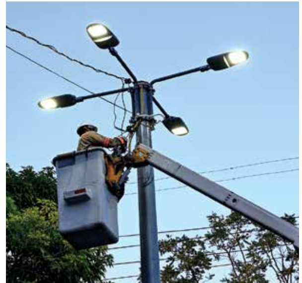
A member of PLD installing some of the 120W LED street lights along the Brian Lara Promenade.
