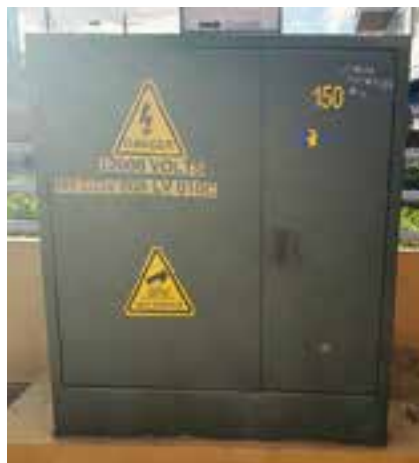
Pad Mounted Transformers
