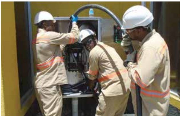
Employees installing cables and other equipment to connect the standby generators.
