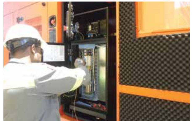
Employees installing cables and other equipment to connect the standby generators.
