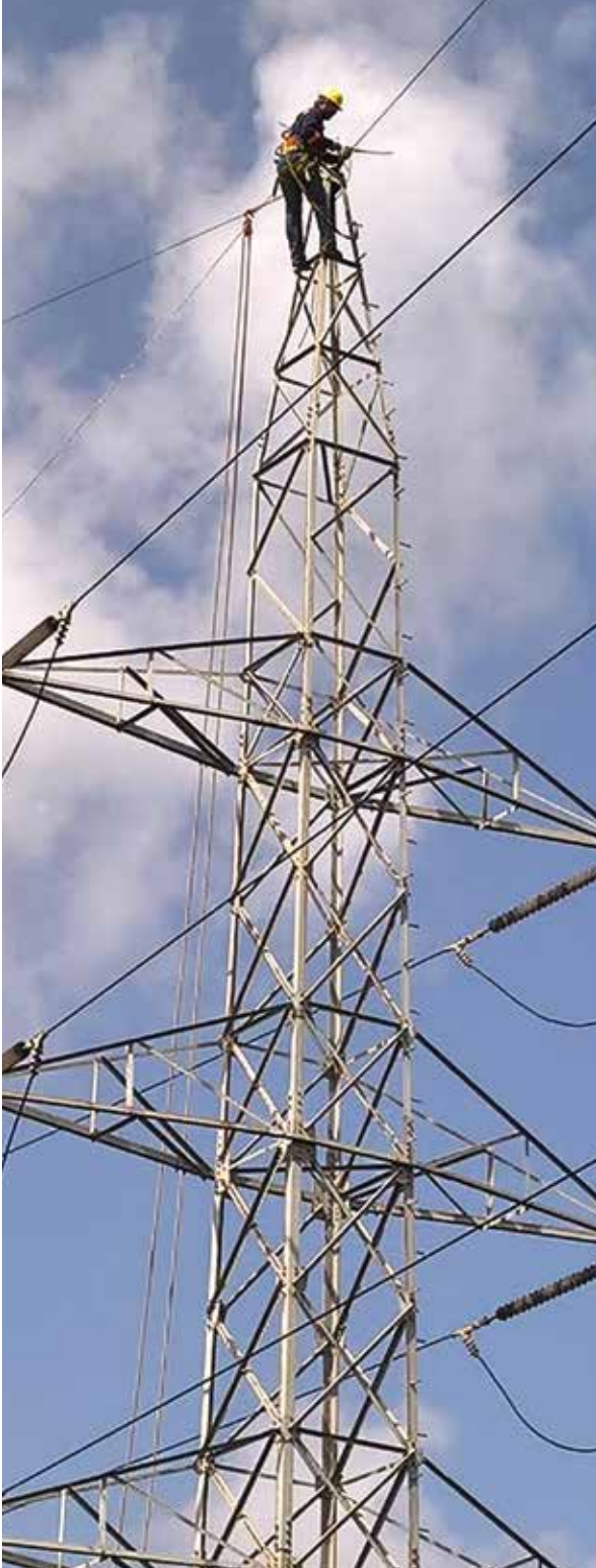
Linesman making preparations to begin the replacement of the aerial conductor.
