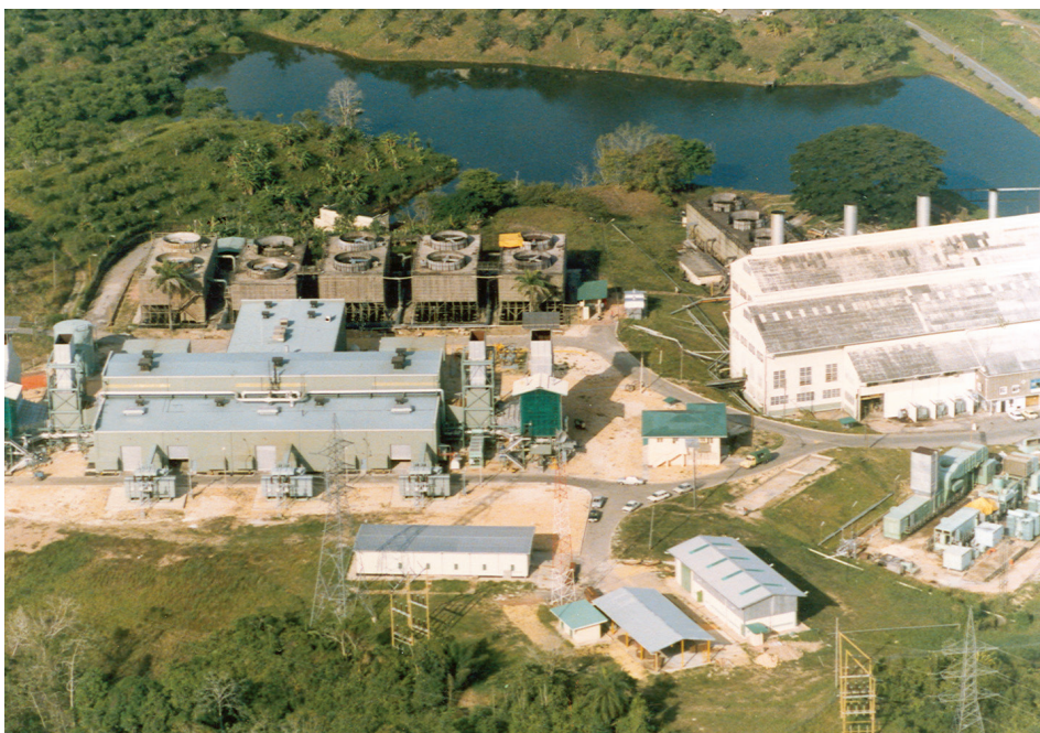
The 186 MW combined cycle generating plant at the Penal Power Station in 1985, built to serve the growing demand of customers.
