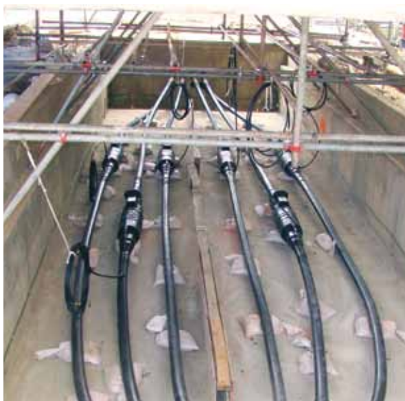
Completed 132 kV joints in JB #1
