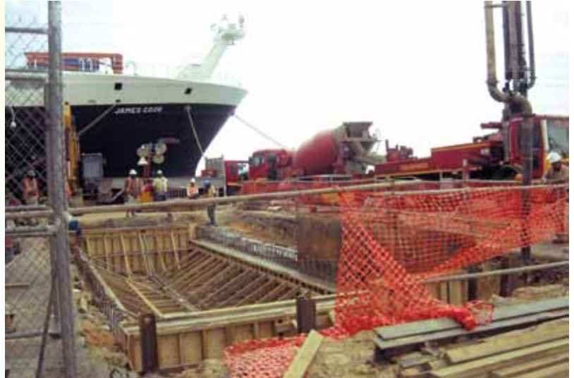
Joint Bay #1 (JB #1) under construction. Location - Port Authority of Trinidad and Tobago (PATT) compound
