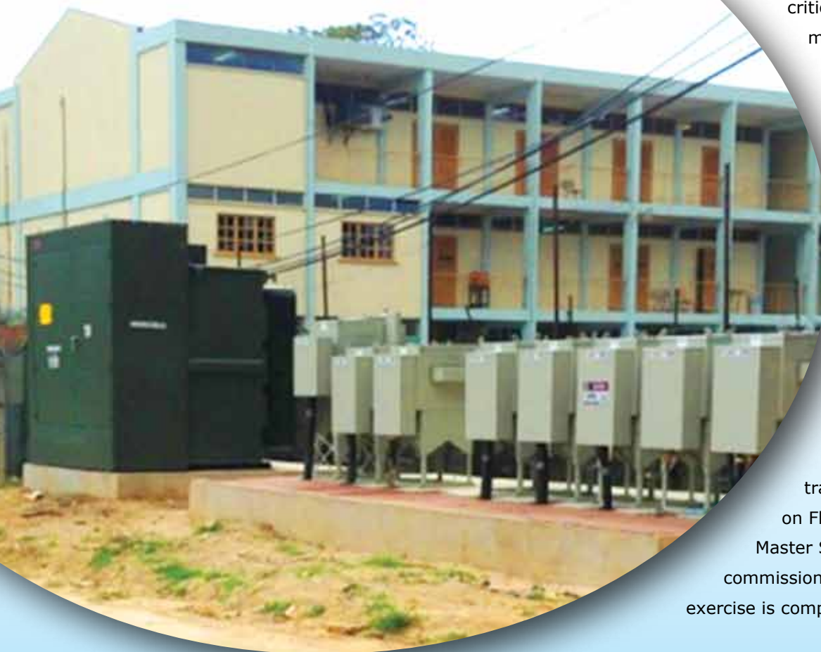
The pad mounted transformer (left) and the ring main unit bank arrangement (right) at the POS General Hospital.
