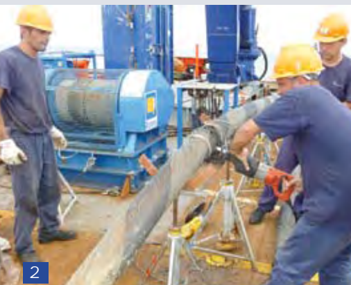
The Italian men from Prysmian cutting the submarine cable using an electric saw.
