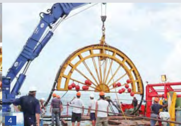
After the jointing operation, the cable bight is lowered on the seabed using a quadrant.
