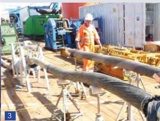
The cable ends aligned for the 2nd joint to be made.
