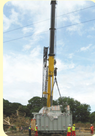
Left: 40/50MVA, 66/33kV Transformer being spotted on its plinth at the Milford Bay Substation extension.
