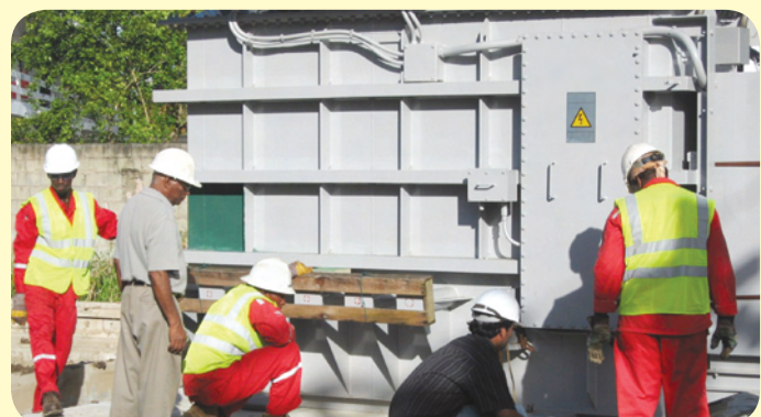
Proper alignment of 12.5/16MVA, 33/12kV Transformer on plinth being verified.
