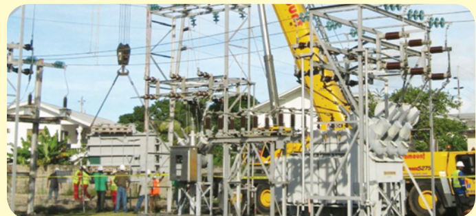
Crane with new 12.5/16MVA, 33/12kV Transformer, towers over existing Milford Bay Substation.
