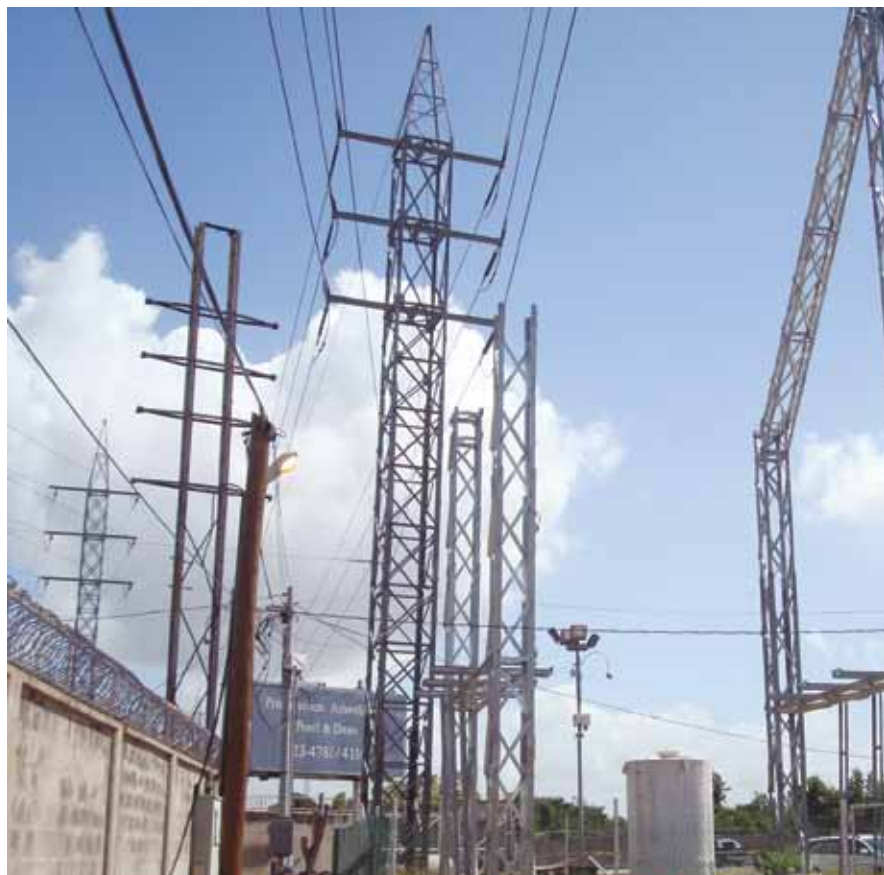
The transition structure at Caricom Jetty off Wrightson Road, which facilitates the transition from overhead lines to underground cables.
