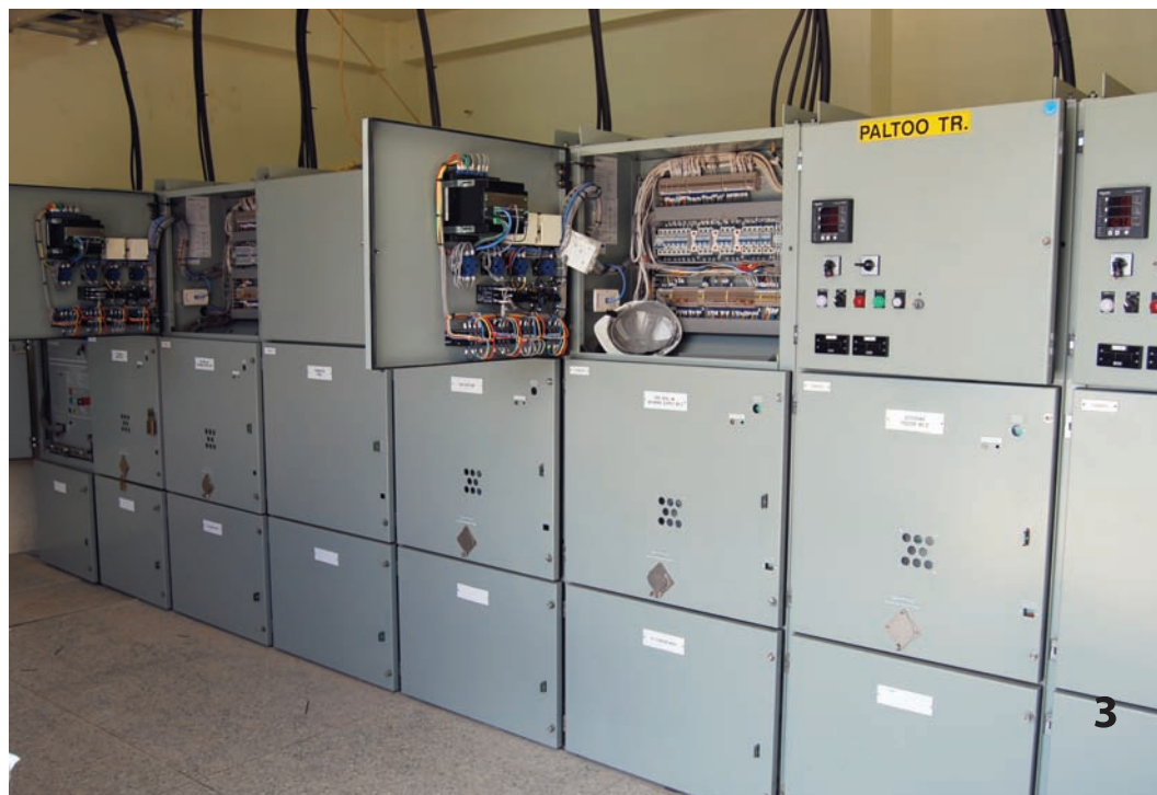
Photos show the Indoor 33 kV SF 6 gas insulated switchgear.
